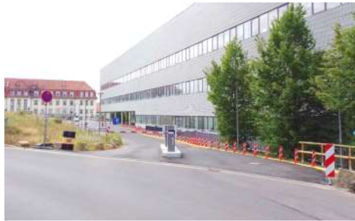
Entrance to RVZ main entry (Building D15)
