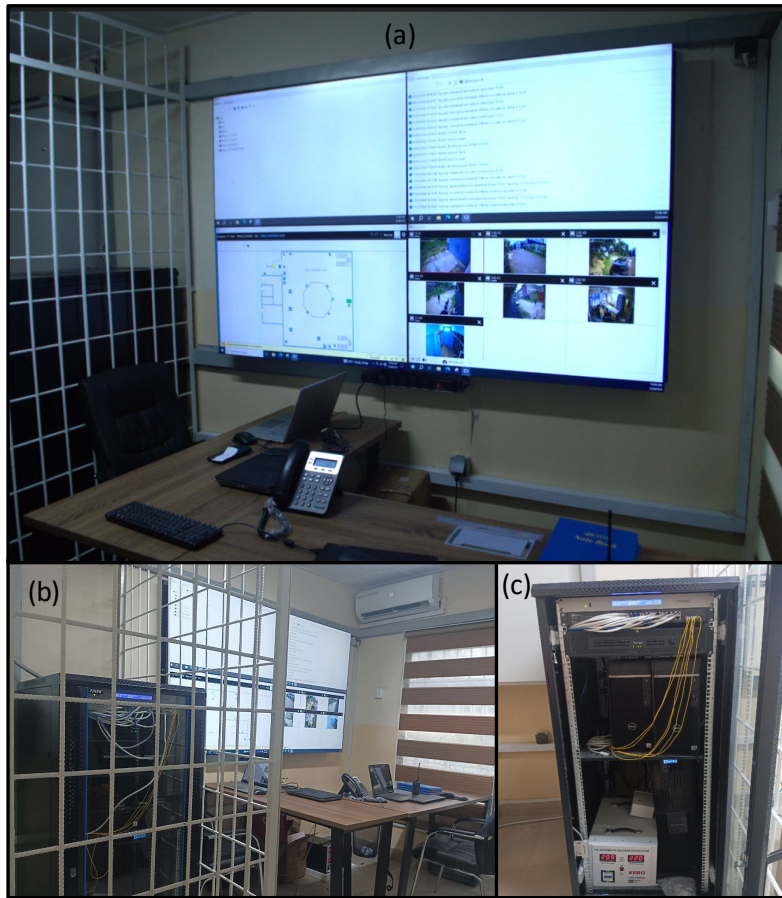
Figure 7: Central Alarm Station monitoring screens (a), secure cage with magnet to secure rack unit (b), rack unit overview (c)
