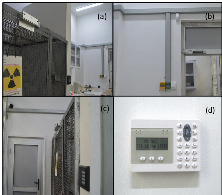
Figure 11: Calibration and Sterilization Lab (a), emergency exit device equipped with motion detector (b), and a cage with magnet protected by an access code (c), disarm keypad and exit button (d)
